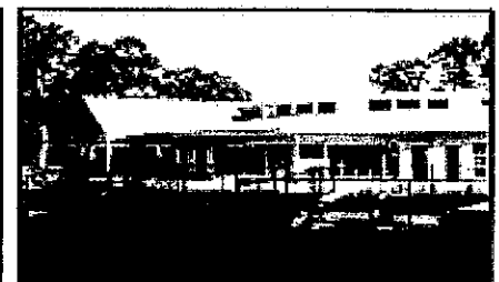
Good Shepard Daycare Center Milford, CT General Contractor, 2009
